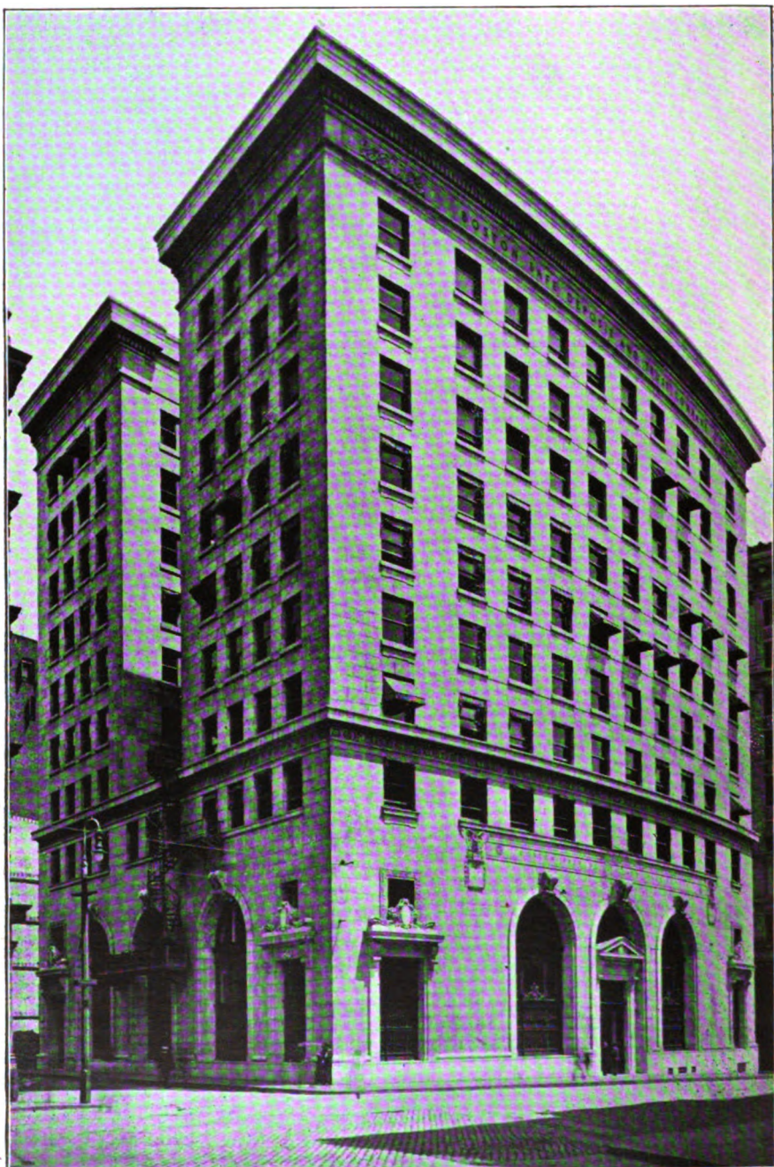
BOSTON SAFE DEPOSIT AND TRUST COMPANY BUILDING Franklin, Devonshire and Arch Streets, Boston
